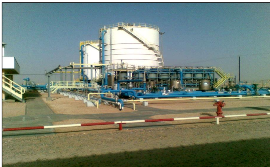
Fig. 2 Farrud main injection station
