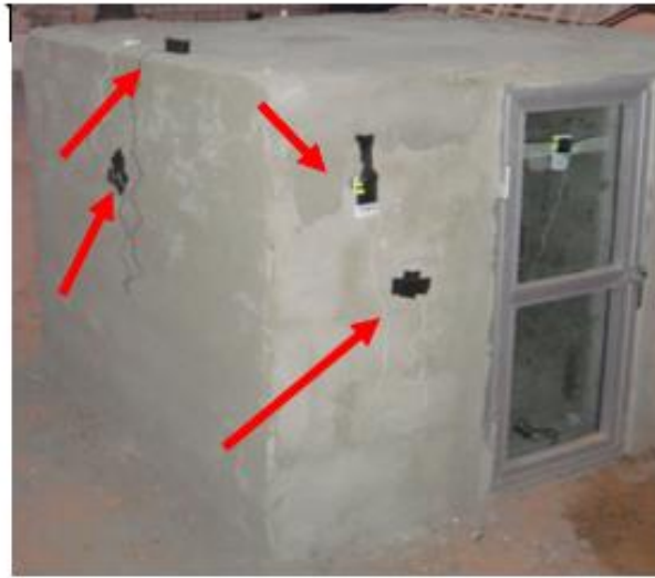
Figure (1) shows the room and temperature sensors.
